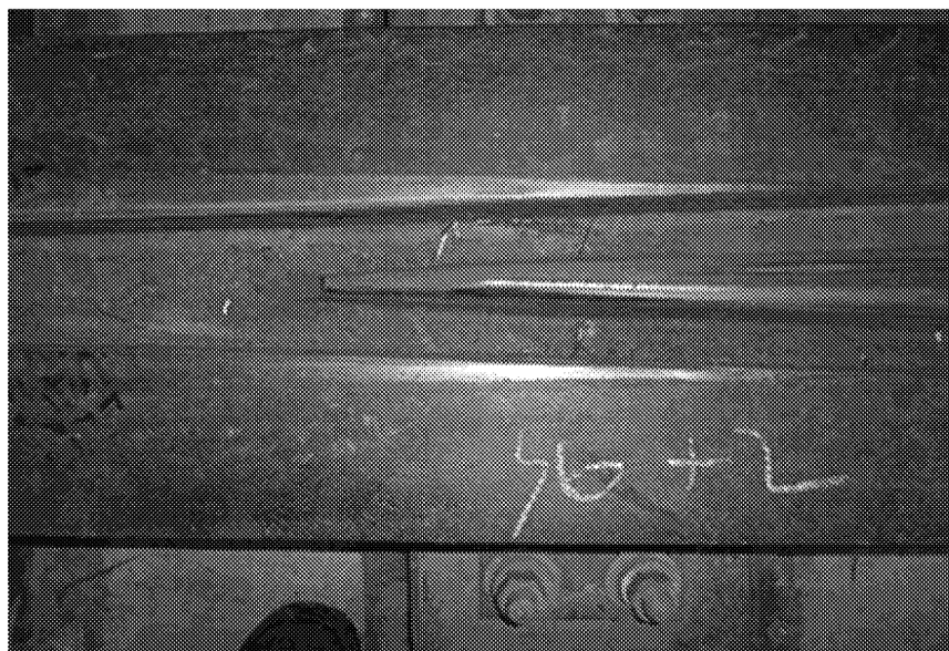
Figure 9: Crossing Wear
