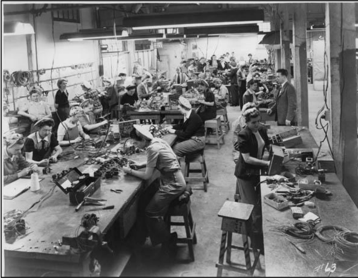
Women soldering and assembling cables for airplanes, Canadian Car and Foundry Co.
