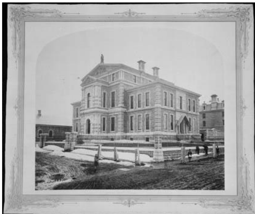
Ottawa Courthouse [ca. 1900] RG 15-90-0-0-59 Public buildings – oversized photographs
