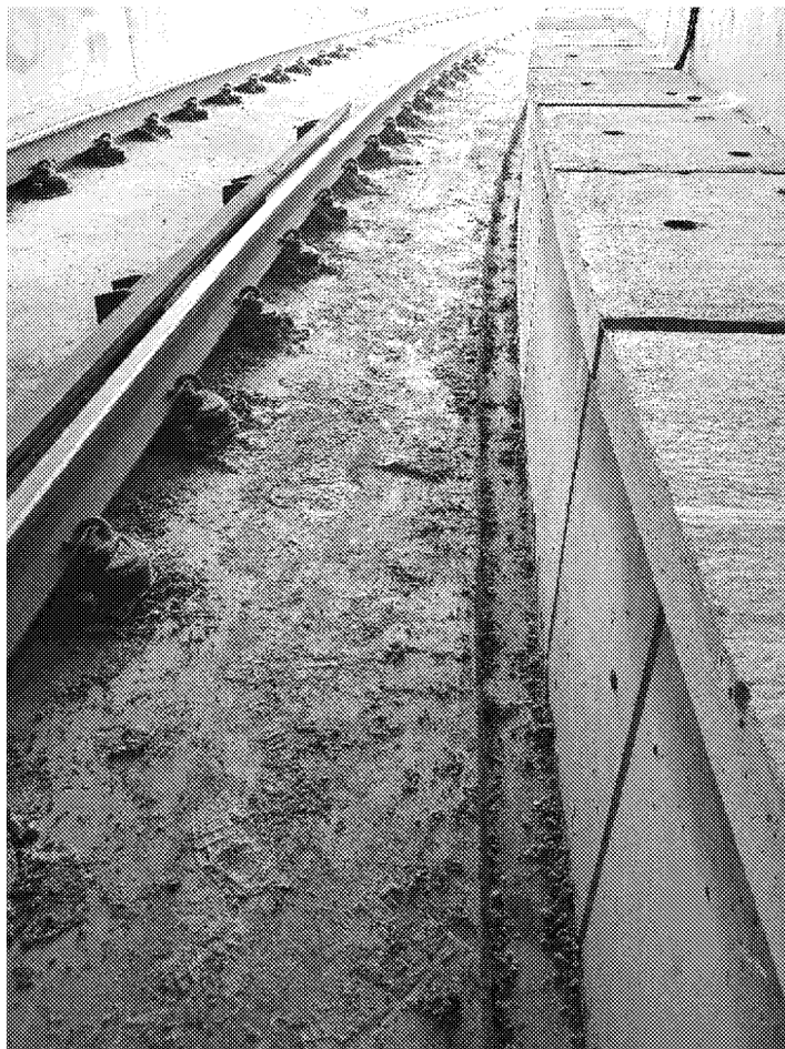
Figure 5.9: Sand in East Connector Portal Tunnel
