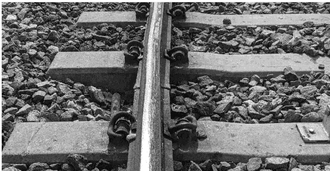
Figure 4.21: Kinks at Weld Location (C19), Including Grease Contamination of the Top of Rail
