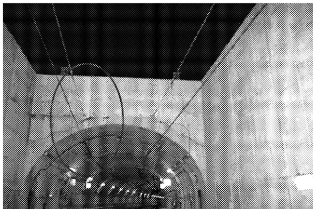
Figure 3.38: Messenger Wire to OCR Jumper Wire
