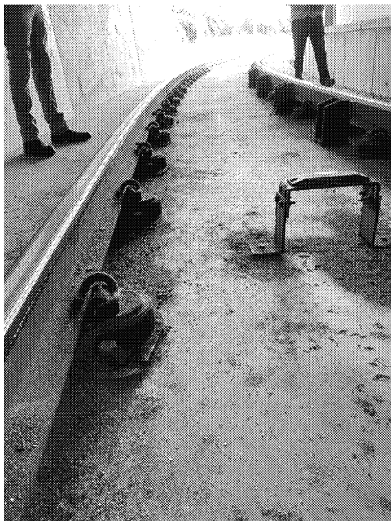
Figure 4.17: Grease Contamination at East Connector
