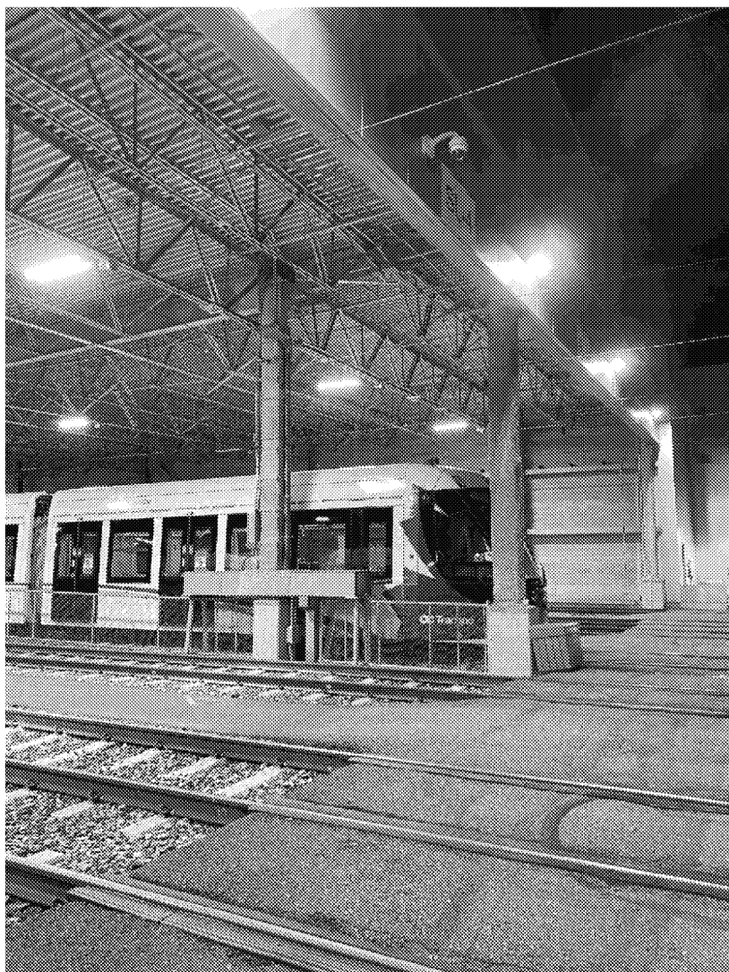
Figure 4.12: Lack of Doors at Storage Shed
