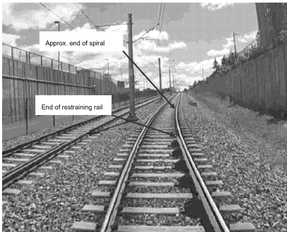
Figure 3.5: Cab footage showing termination of the restraining rail within a spiral
