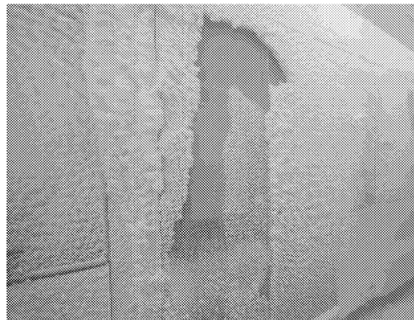
Figure 33 - LMC2 Door Snow Accumulation
