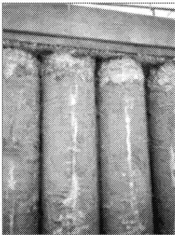
Figure 5.3.3A | Typical Secant Pile Support
