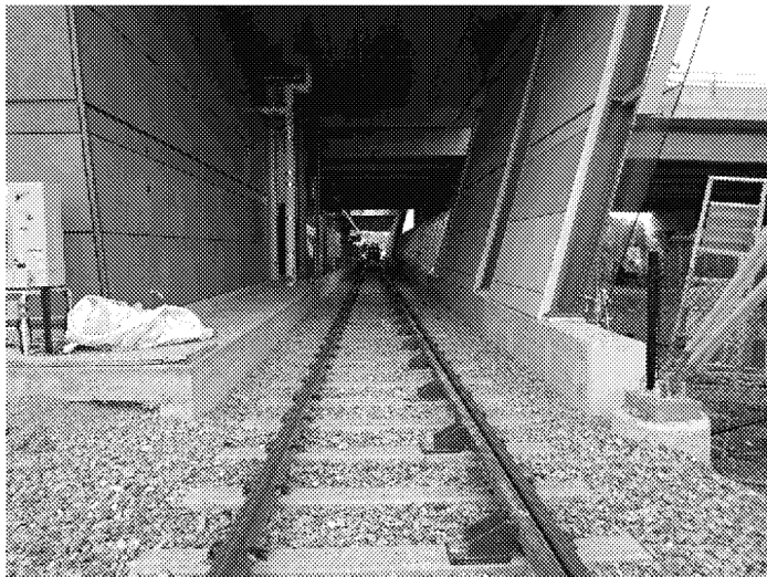
Photo 15 (left): Restraining rails in Pimisi west bound platform. Photo 16 (right): Restraining rails in Pimisi east bound platform.
