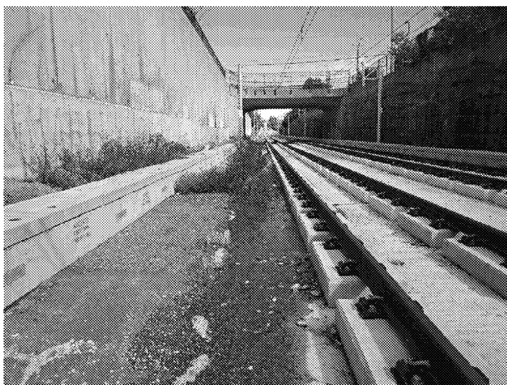
Photo no. 13: Excessive vegetation growth along side the track at 98km 550m, west bound side.
