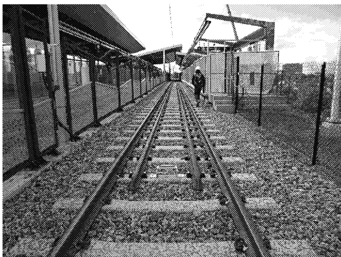
Photo no. 17 (left): start of Jordan rail protection west bound into Bay View station.
