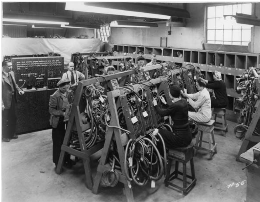
Women wiring the main distribution panels for airplanes, Canadian Car and Foundry Co. 1945, Fort William (Ont.) Canadian Car and Foundry Collection Reference Code: C 190-3-0-0-42 Archives of Ontario, I0002964
